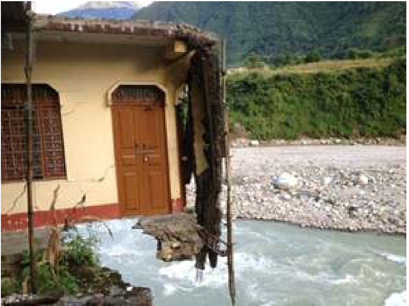
(Top) Maniram's home destroyed during flash floods following the Uttarakhand disaster
